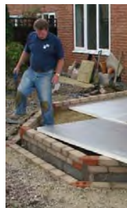
Insulation installed
