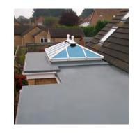
in the build up. Pre-form GRP edge trims are fitted to finish the sides, then our installers lay a hard wearing, heavy duty Britelite GRP laminate onto the surface, as standard.
